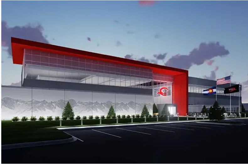
Image shows a rendering of the new QTS Aurora-Denver Campus currently under construction.
