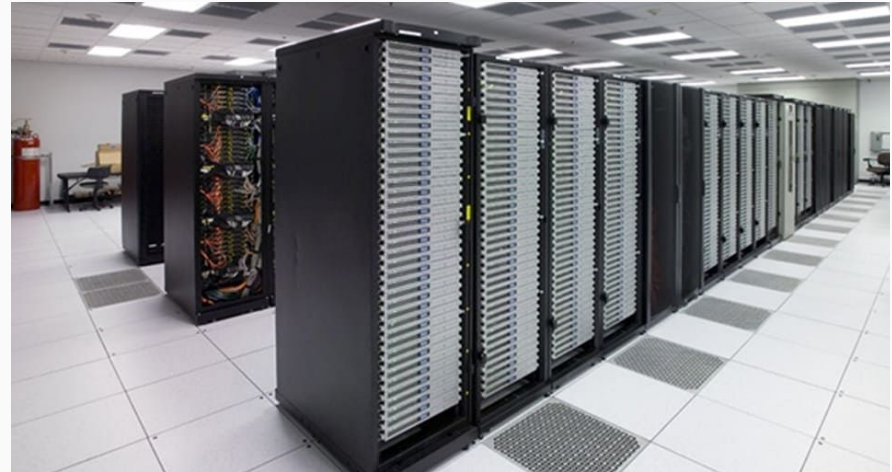
Image shows an example of standalone, prefabricated data center cabinets.
