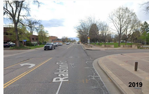
Ralston Road Ph 2 (Ammons)– (Before and After)
