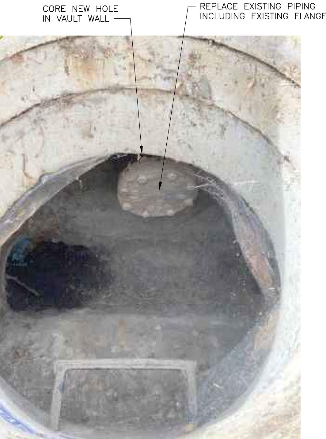
PHOTO INSIDE OF CARR ST. DRAIN VAULT (SHEET C-2)
