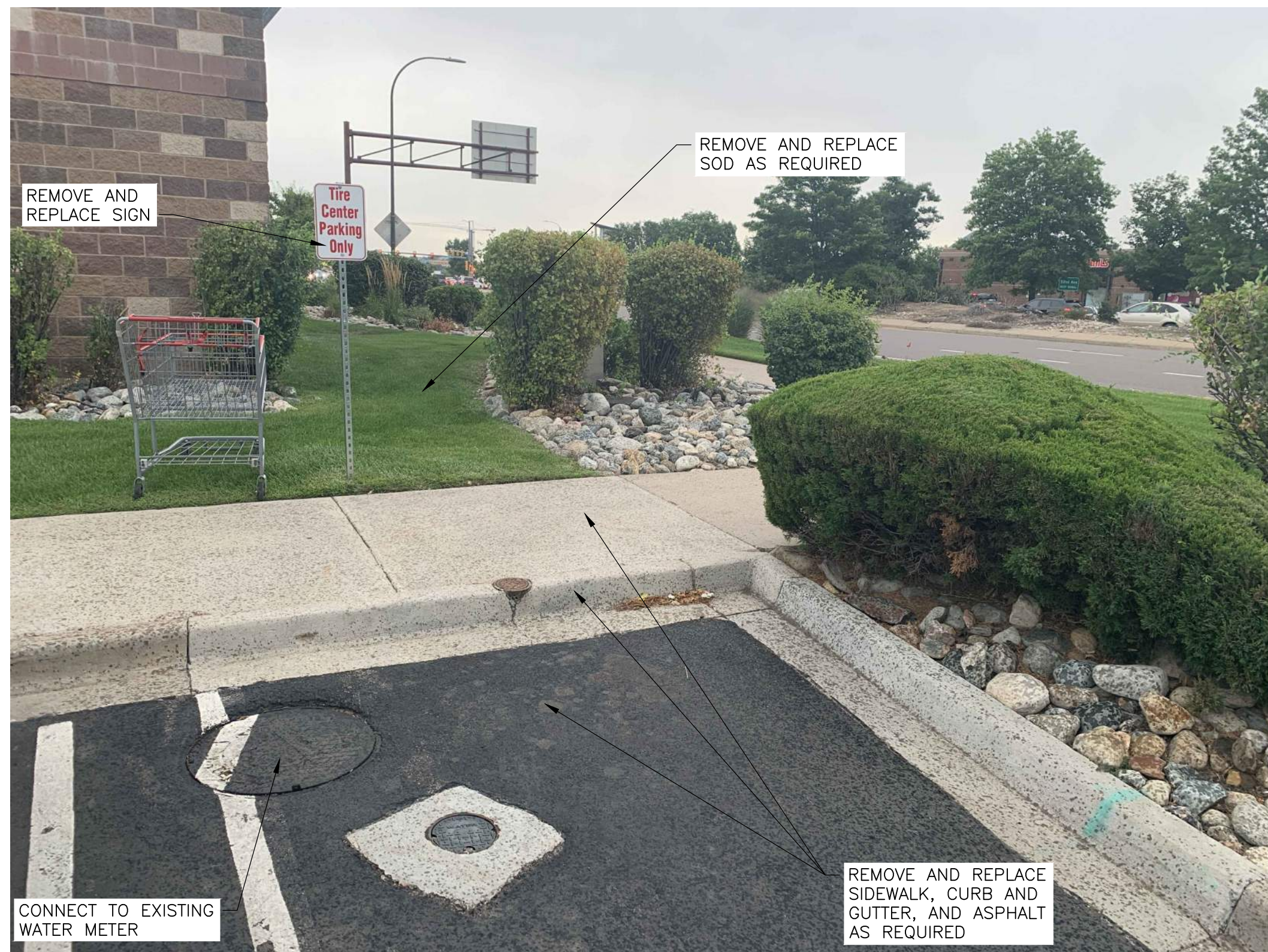
COSTCO METER RECONNECTION
