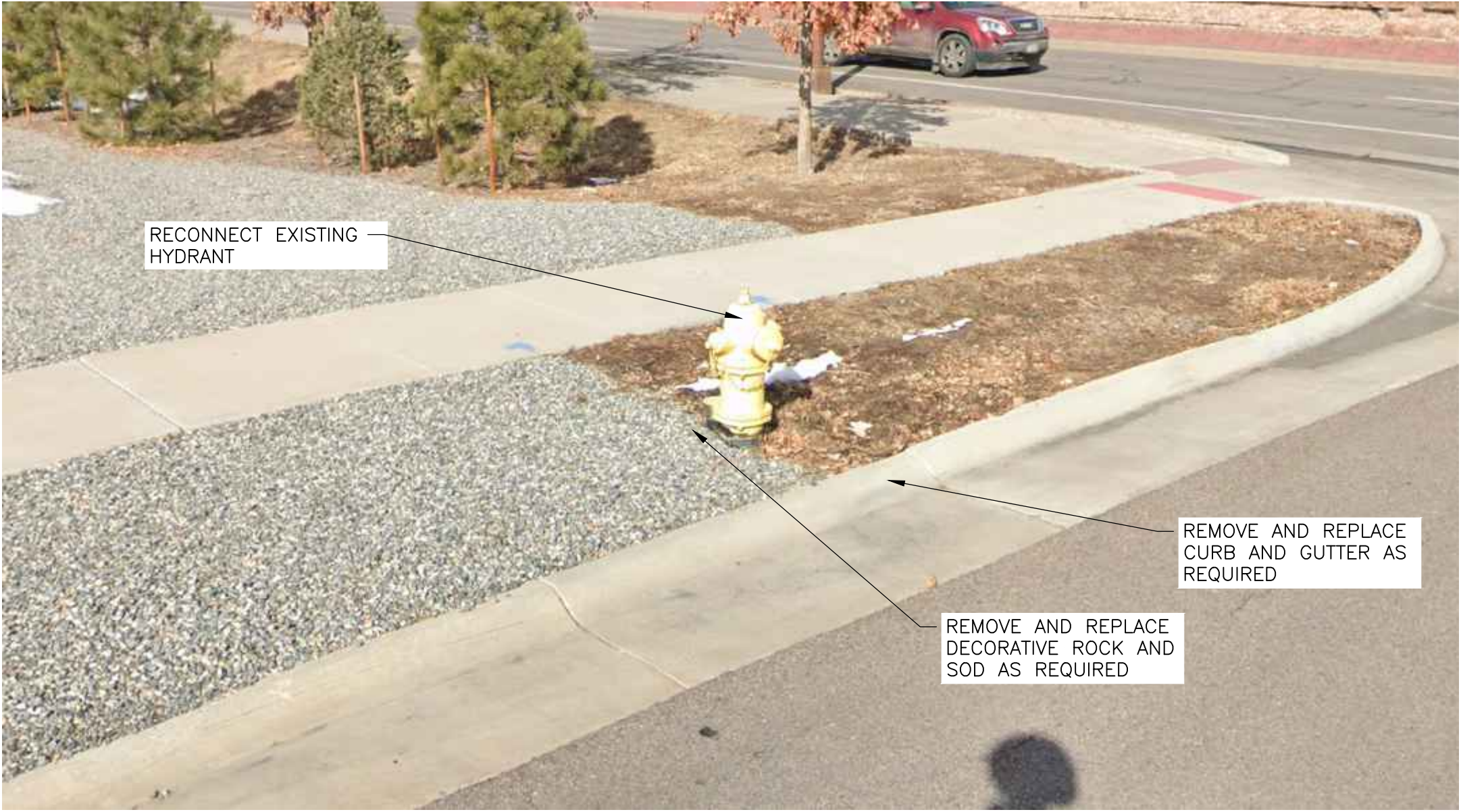
HOLLAND CT. HYDRANT CONNECTION DETAIL E NTS
