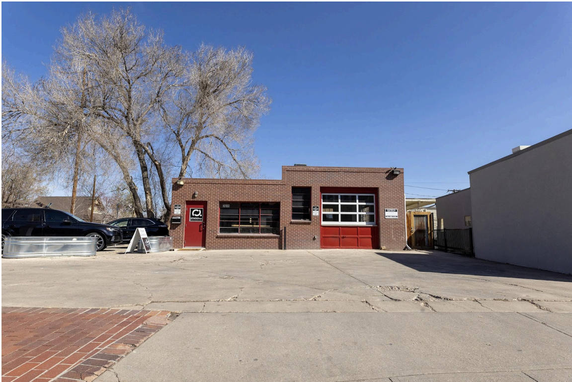
Existing Condition (south elevation) 2024
