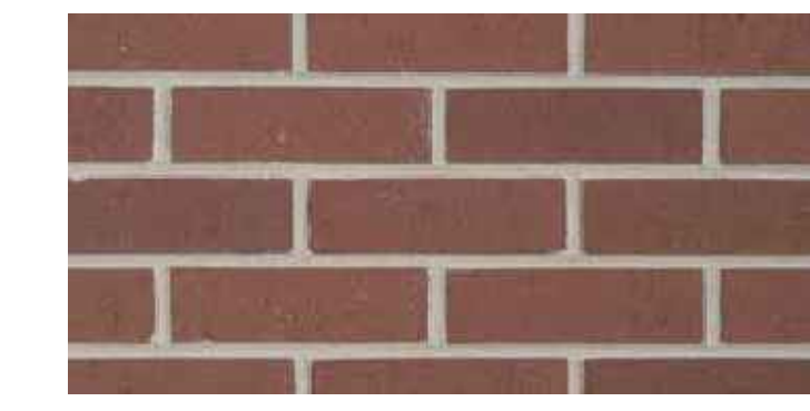
BRICK AT WEST SITE WALL
