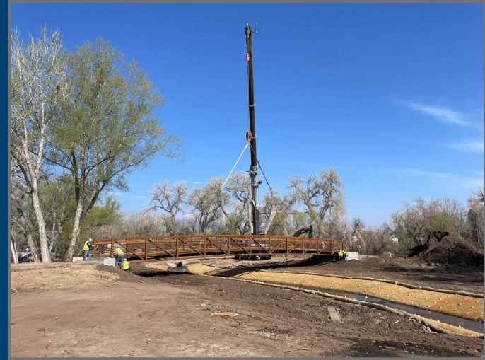
Ralston Creek at the Croke Canal crossing Expected completion Fall 2025
