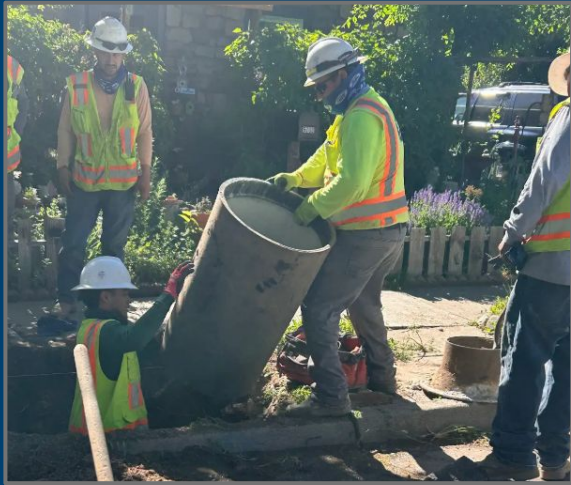
Lead Service Replacement project
