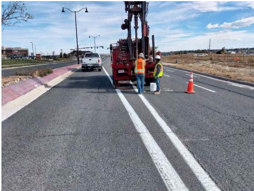
Photo 2. View looking north at drilling operations on Indiana Street.
