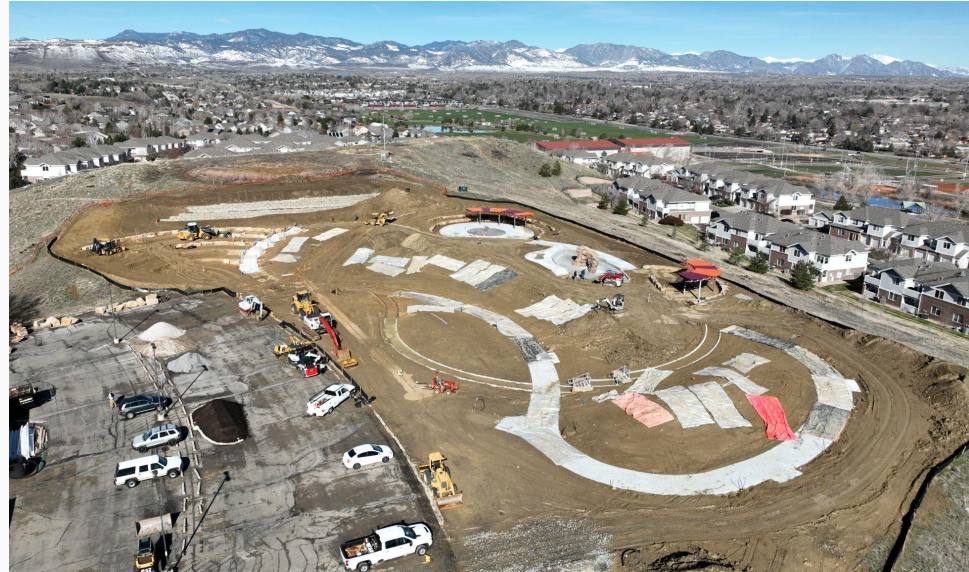
Aerial image of construction progress : March 2024
