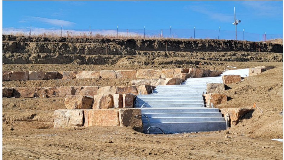
Construction photo January 2024
