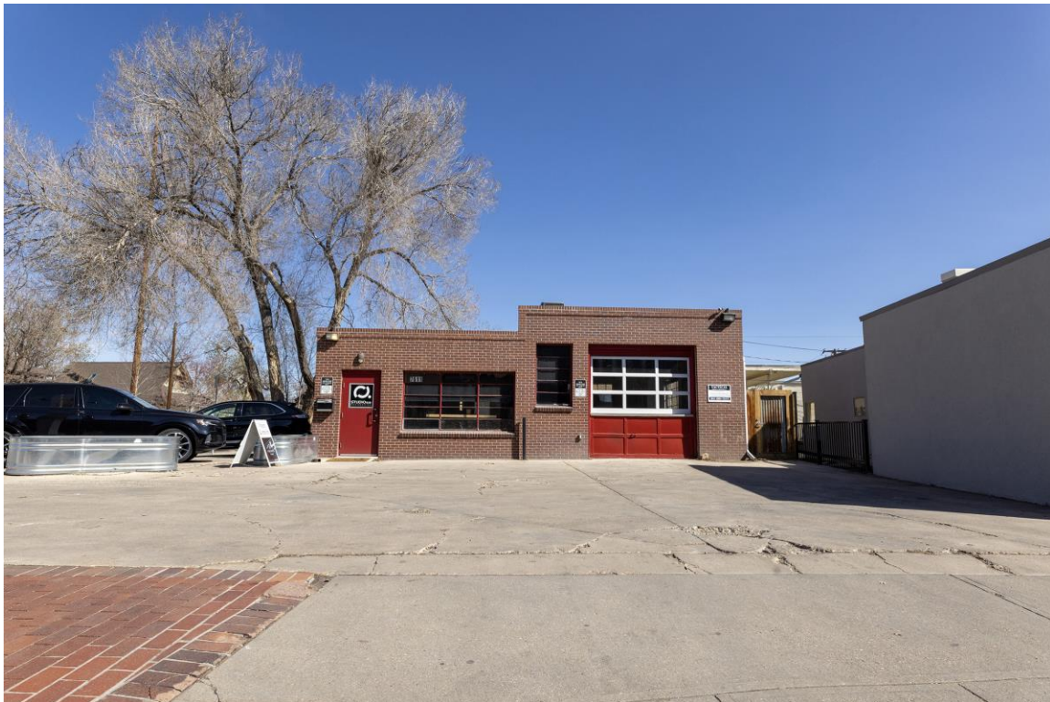
Existing Condition (south elevation) 2024
