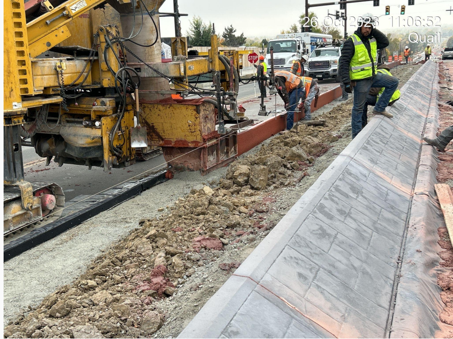
New Median Under Construction
