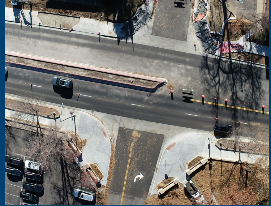
11/17/2023 (After final paving)
