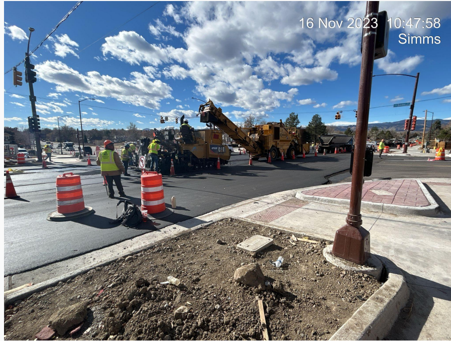
Paving Simms Intersection
