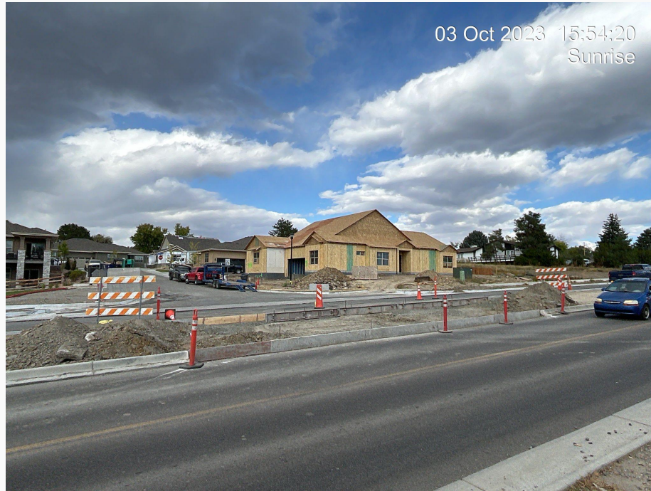
Sunrise Village Entrance During Construction
