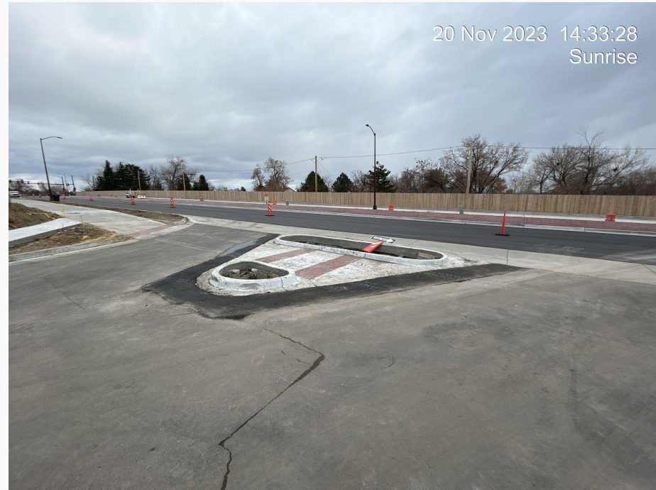
Sunrise Village Entrance Completed
