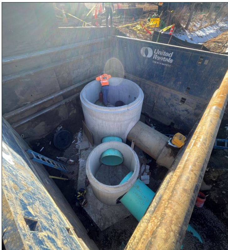
Deep excavation for the installation of two manholes with 36" sewer pipe required specially engineered shoring.
