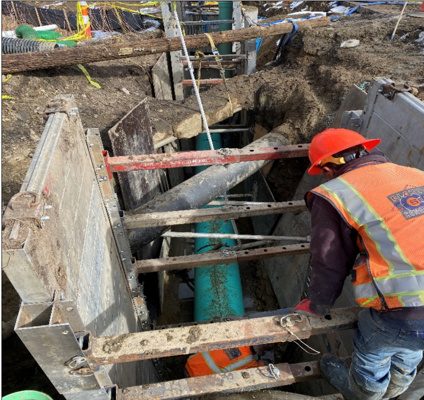
Trenching and installing multiple manholes and a 27" sewer line crossing a high-pressure 16" gas line, a concrete encased phone bank, fiber optics, and other utilities required careful planning of shoring equipment. Mitigation of an abundance of ground water in the trench was required during the entire process.
