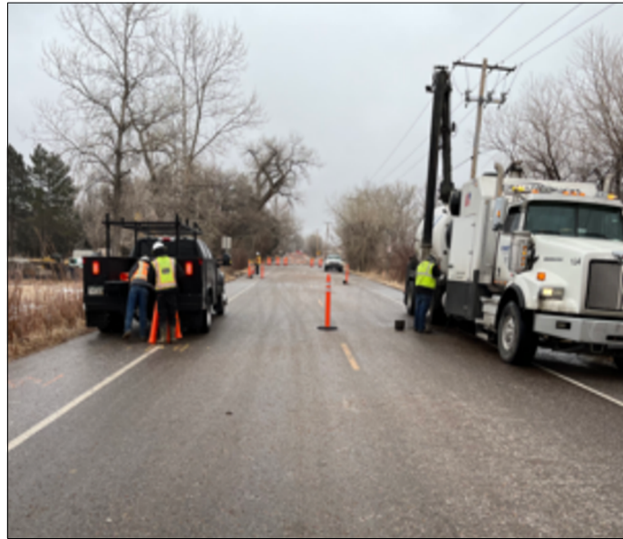
Potholing using a vac-truck was vital for worker safety and protection of a high-pressure gas line and other utilities.
