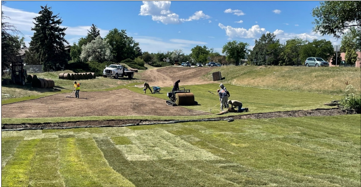
Waterway and Retention Basin Reclamation: Reseeding and landscape repair along roadways and retention basin was required.
