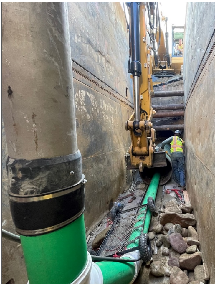
High volume of groundwater was present at box culvert boring site. Constant groundwater mitigation was required through the boring process.
