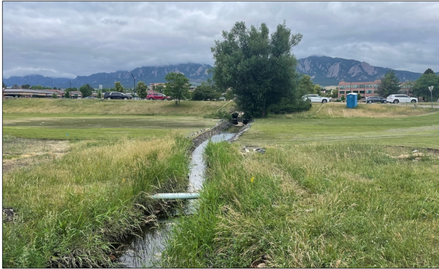
East Boulder Creek Ditch: This was an active waterway especially during the spring runoff season. Careful SWPPP mitigation and a temporary 18" bypass carrier pipe was used while Native Sun installed a sewer line underneath the waterway and replaced the concrete base of the ditch.
