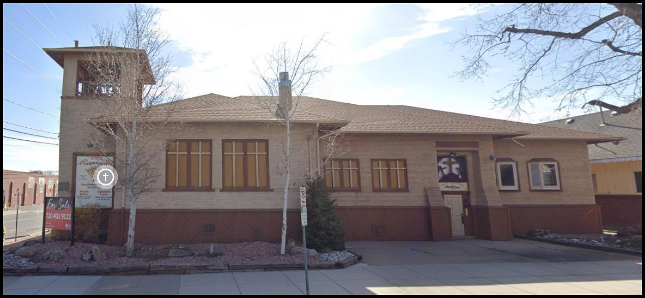
Existing West Façade (Google Streetview, April 2022)
