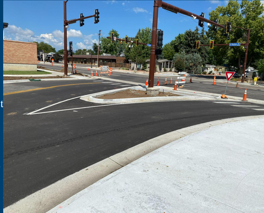
Balsam and Ralston Rd intersection with new pavement
