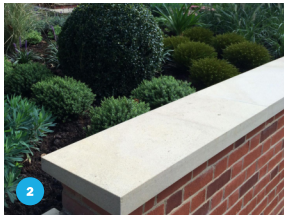
LOW BRICK RETAINING WALLS W/ SANDSTONE CAPS
