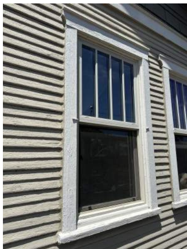
Existing fiberglass windows.
