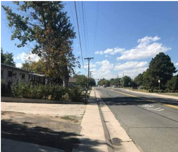
Undersized sidewalk on 60th Avenue.
