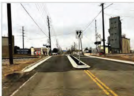
120th Avenue Railroad Crossing Without Sidewalks (pre-construction)
