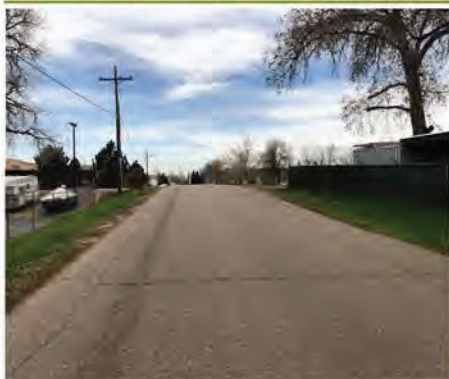
Upah Street Pre-Construction
