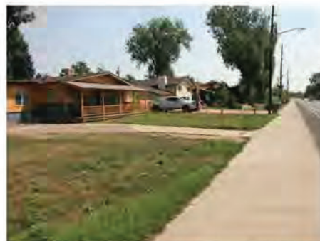
Properties east of Miller Street impacted by underpass cut
