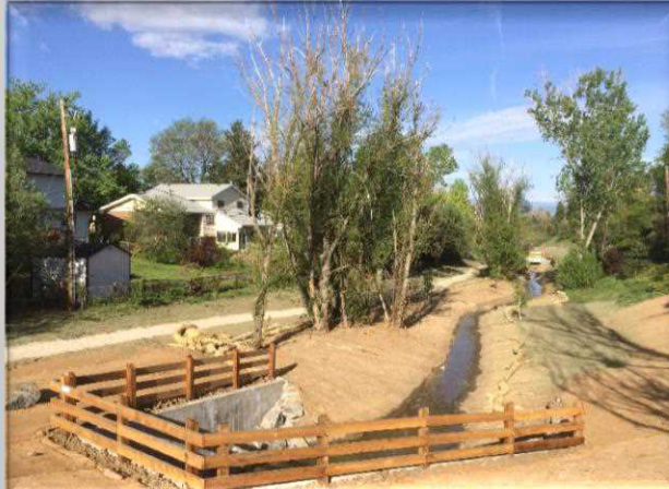
* Little Dry Creek Drainage Improvements
