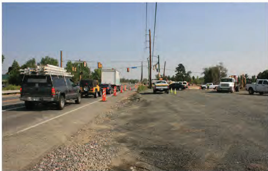
Intersection Improvements Under Construction - August 2018
