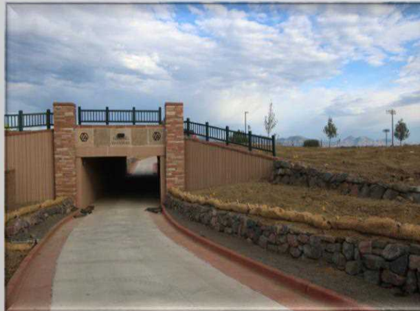
* Kipling Underpass-Trail Extension
