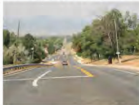
Vertical break west of Quail Street
