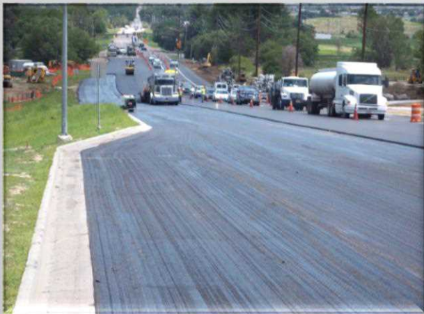
* 104 th Avenue Widening
