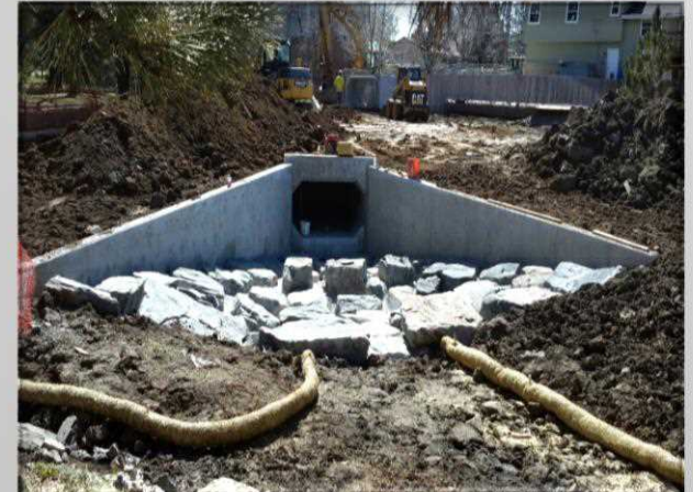
* Walnut Hills Drainage Improvements
