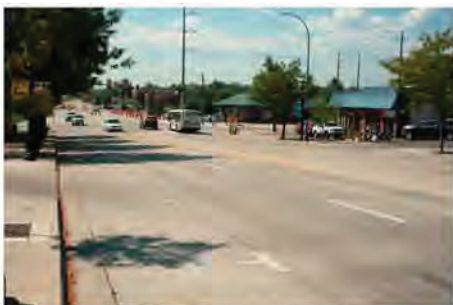
US 287 Main Street, Ken Pratt Boulevard to 3rd Avenue, City of Longmont
