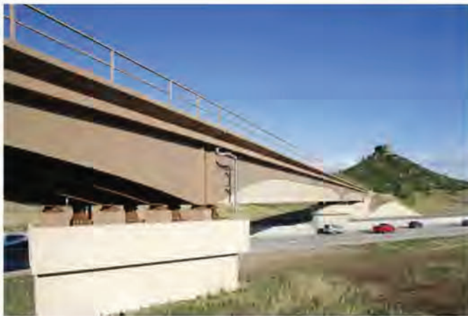
HDR's High Skew Railroad Bridge, Castle Rock, Colorado
