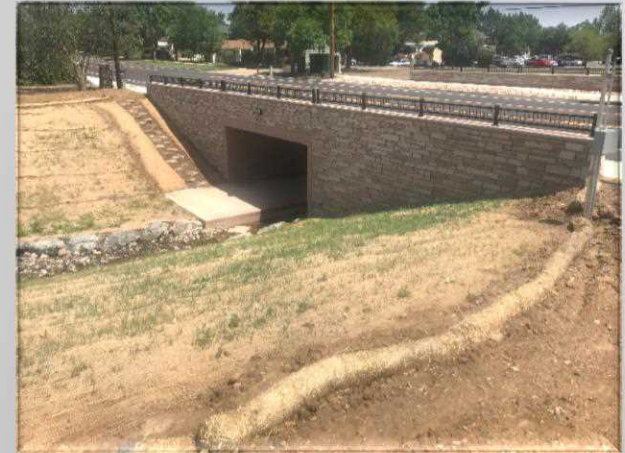
*111 th Street Drainage Improvements
