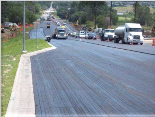
* 104 th Avenue Widening
