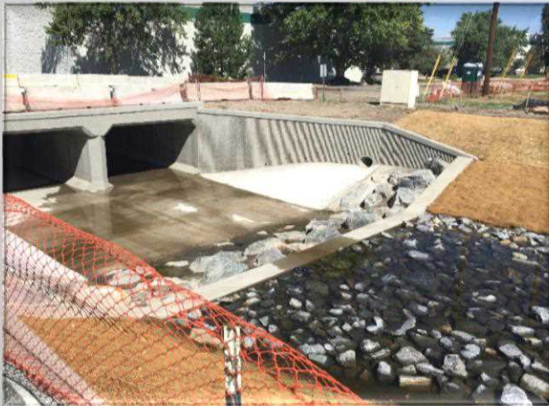
* Baranmor Ditch Improvements
