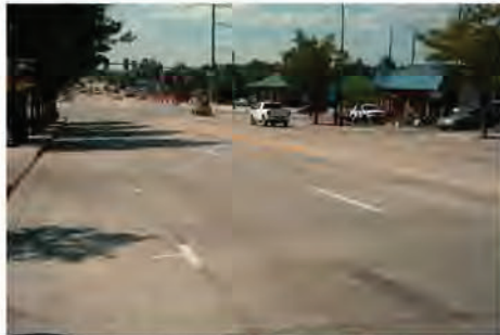
US 287 Ken Pratt Boulevard Reconstruction, City of Longmont
