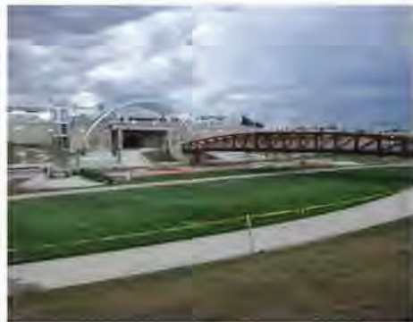
Little Dry Creek Transit Station Pedestrian Bridge, City of Westminster and UDFCD
