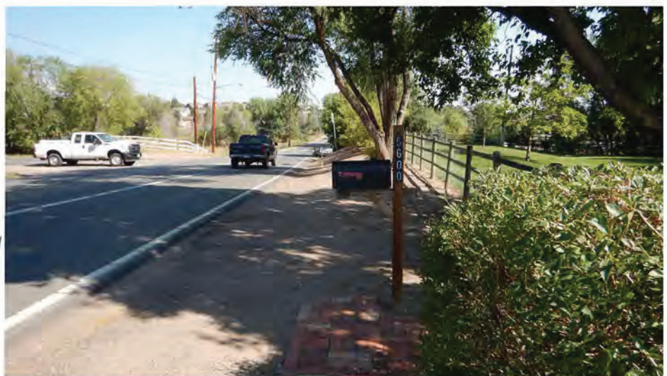
Existing Roadway to be Reconstructed to Four-Lanes with Bike Lanes and Sidewalks
