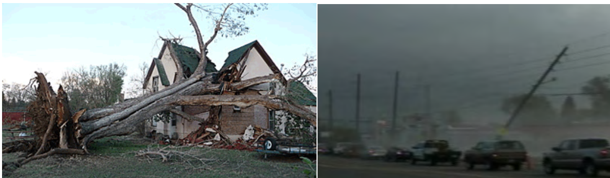
Figure 4-56 July 20, 2009 Damage in Wheat Ridge
