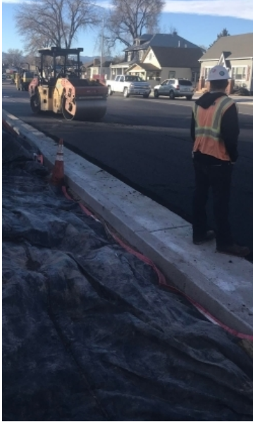
TOP LIFTS PAVED (Completed May 10th)
