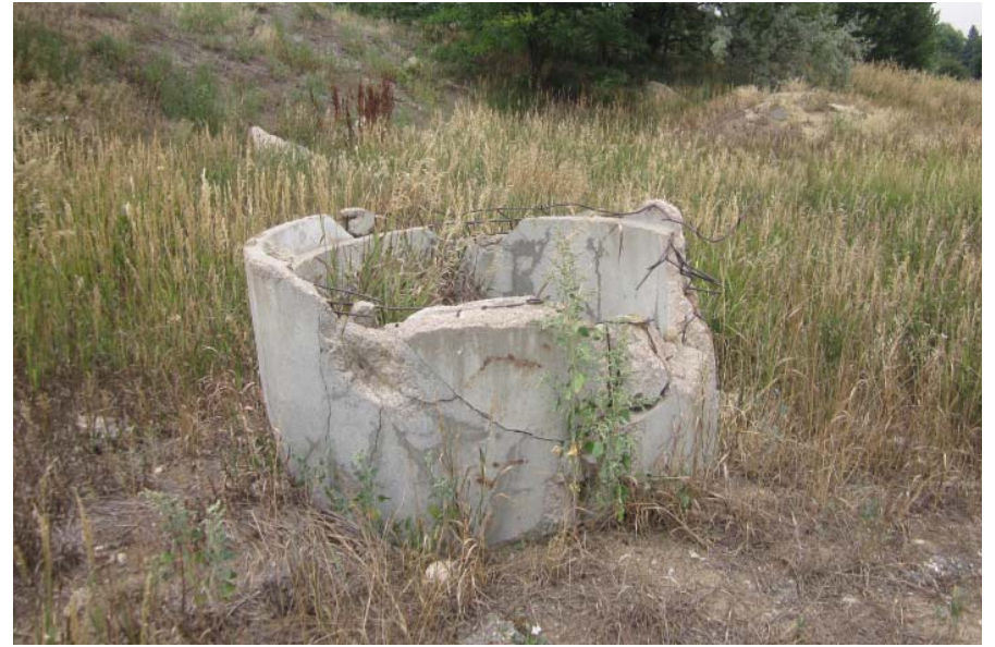
CONCRETE DEBRIS DOTS PARTS OF THE SITE
