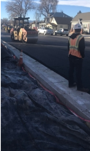
BASE LIFTS PAVED (Completed Dec. 11)
