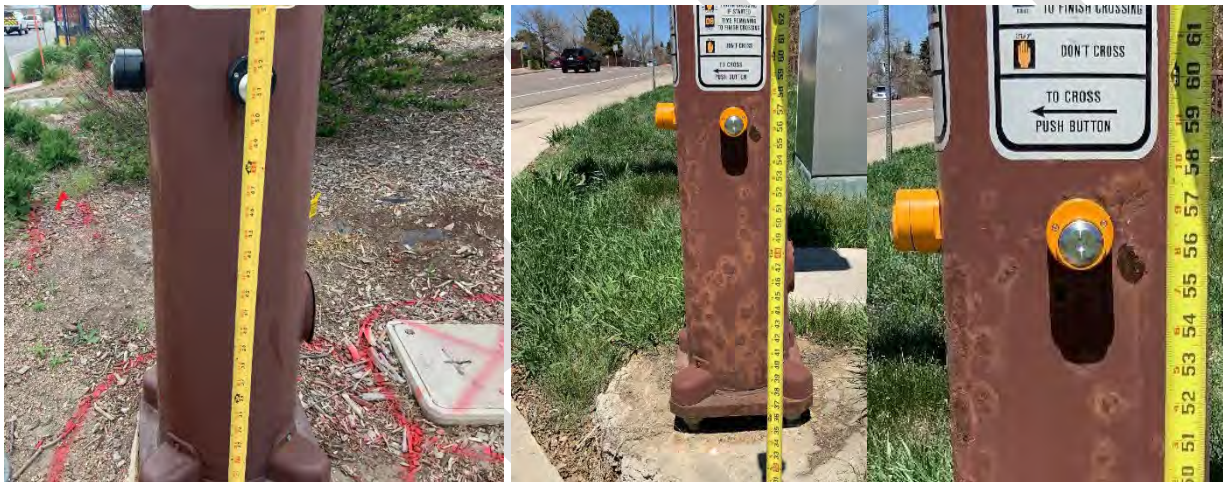
Figure 2.6.1.2(g) Typical Observation: Pedestrian control is too high. [PROWAG R406. ]
