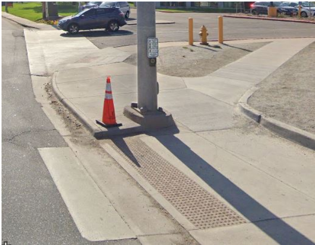
Figure 34 Pedestrian control is higher than 48 inches.
