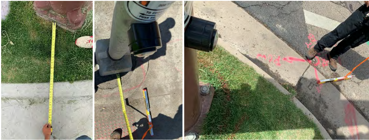
Figure 2.6.1.2(g) Typical Observation: Pedestrian control is too high. [PROWAG R406. ]
