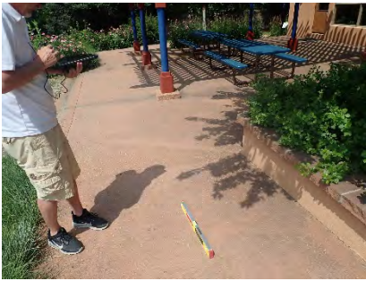
Figure 2.4.1.3(d) Typical Observation: Accessible routes with slopes too steep: [ADA Standards 403.3 ]
