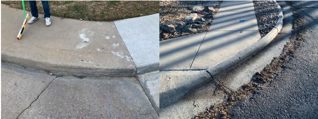
Figure 2.6.1.3(f) Typical Observation: Turning space at top of curb ramp is too narrow/obstructed. [ PROWAG R304.2.1. ]
