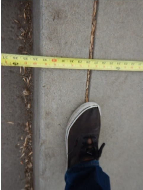
Figure 21 Measurement shows the sidewalk is 28 inches wide.
