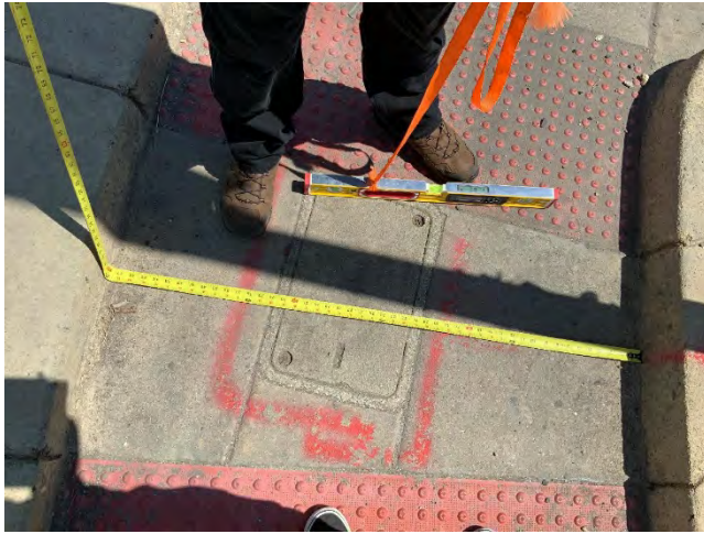
Figure 2.6.1.3(j) Typical Observation: Pedestrian access route (PAR)/pedestrian street crossing not 60 inches wide minimum within pedestrian refuge island. [ PROWAG R302.3.1. ]
