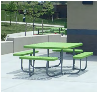
Figure 2.5.1.1(d) Typical Observation: Insufficient knee clearance at picnic table. [ADA Standards 306.3.3. ]
