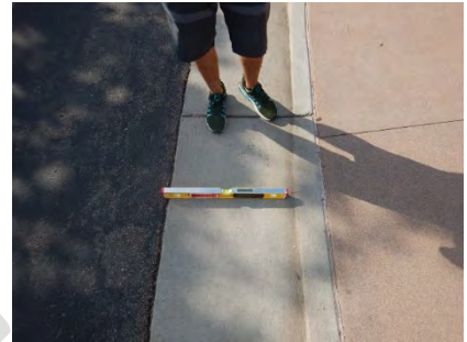
Figure 2.4.1.3(a) Typical Observation: Curb ramps with slopes too steep: [ADA Standards 406. ]
