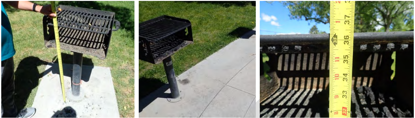
Figure 2.5.1.1(c) Typical Observation: 48 inches of clear ground space is not provided on all usable sides of grill. [ABAAS (ODA) Table 1011.2.1 ]
