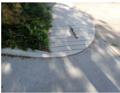
Figure 2.4.1.3(a) Typical Observation: Curb ramps with slopes too steep: [ADA Standards 406. ]
