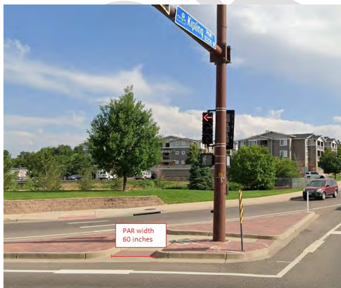
The clear width of pedestrian access routes within the pedestrian refuge island at W 58 th Ave & Kipling Parkway.
