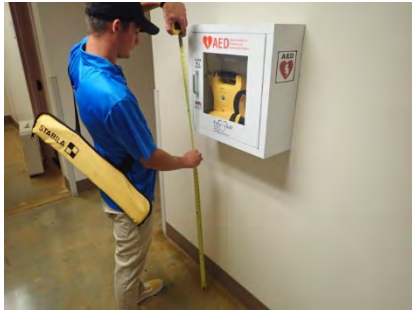
Figure 2.4.1.1(b) Typical Observation: Protrusions throughout facilities: [ADA Standards 307. ]
