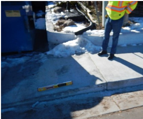
Figure 24 Data collector measuring the running slope of the sidewalk at a driveway.
