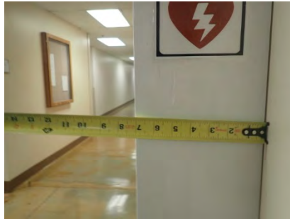
Figure 2.4.1.1(b) Typical Observation: Protrusions throughout facilities: [ADA Standards 307. ]
