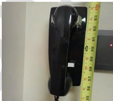
Figure 2.4.1.1(c) Typical Observation: Operable parts above required reach range: [ADA Standards 308. ]
