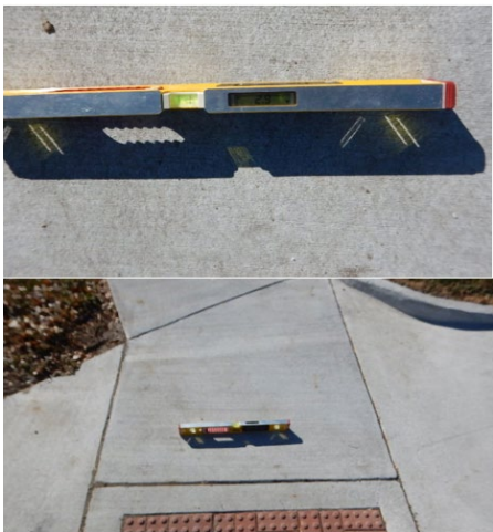
Figure 5 Measurement shows the cross slope of this curb ramp is 2.9%
