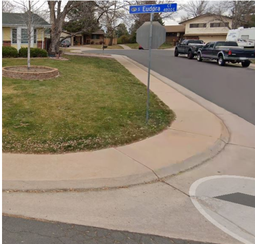
Figure 6 No curb ramp at corner.
