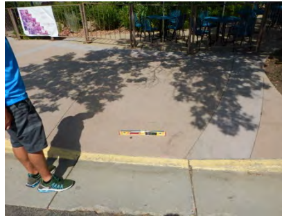
Figure 2.4.1.3(a) Typical Observation: Curb ramps with slopes too steep: [ADA Standards 406. ]
