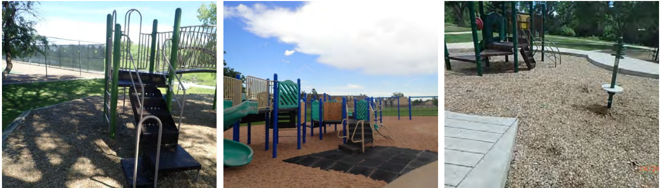
Figure 2.5.1.3(c) Typical Observation: Play area has no ground level play components on an accessible route. [ADA Standards 240.2.1.1, 1008.4]
