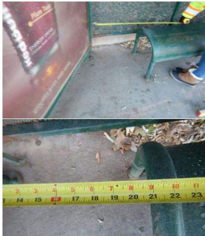
Figure 30 Measurement shows clear space adjacent to bench is less than 30 inches wide.
