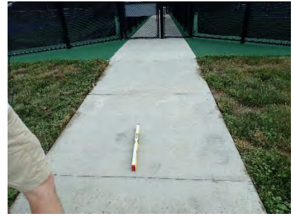
Figure 2.4.1.3(d) Typical Observation: Accessible routes with slopes too steep: [ADA Standards 403.3 ]
