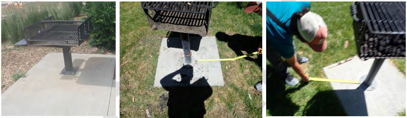
Figure 2.5.1.1(c) Typical Observation: 48 inches of clear ground space is not provided on all usable sides of grill. [ABAAS (ODA) Table 1011.2.1 ]
