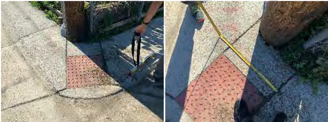
Figure 2.6.1.3(f) Typical Observation: Turning space at top of curb ramp is too narrow/obstructed. [ PROWAG R304.2.1. ]
