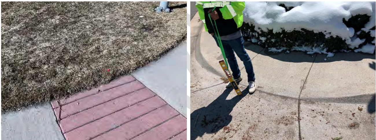
Figure 2.6.1.3(d) Typical Observation: Curb ramp has no turning space at top. [PROWAG R304.2.1. ]
