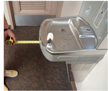
Figure 2.4.1.1(b) Typical Observation: Protrusions throughout facilities: [ADA Standards 307. ]
