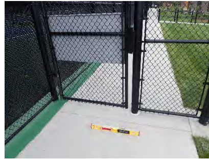
Figure 2.4.1.3(d) Typical Observation: Accessible routes with slopes too steep: [ADA Standards 403.3 ]
