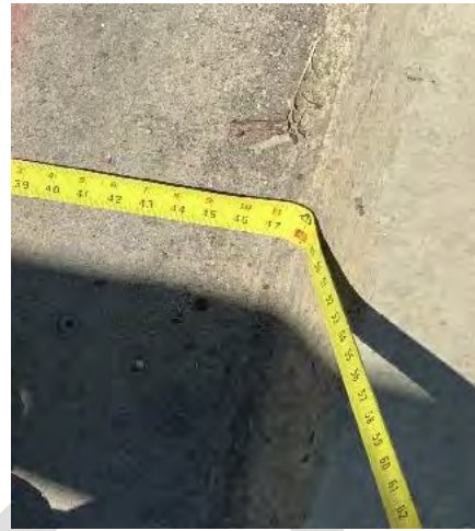
Figure 2.6.1.3(j) Typical Observation: Pedestrian access route (PAR)/pedestrian street crossing not 60 inches wide minimum within pedestrian refuge island. [ PROWAG R302.3.1. ]
