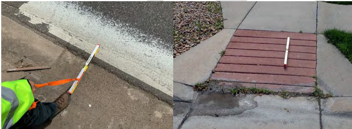
Figure 2.6.1.2(d) Typical Observation: Detectable warning surface not provided on curb ramp. [PROWAG R208 and R305 .]
