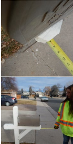
Figure 23 Data collector measuring a mailbox that protrudes nearly 7 inches into the clear width of a sidewalk.
